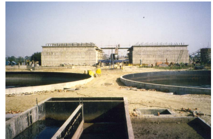
Construction of Kanpur UASB reactors.
